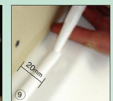
9 Lay a line of Sealux-N on ledge using finger as guide
