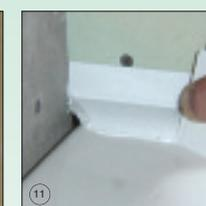
11 Remove excess Sealux-N on ledge (if any)
