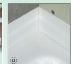
12 Ensure Sealux-N fuses across joints inside strips
