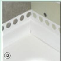
12 Ensure Sealux-N fuses across joints inside strips
