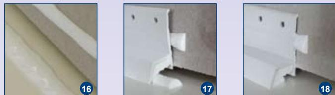
15-18 15. On ledge to receive the first strip, using finger under nozzle as support and fingertip against wall as guide, lay an 8mm line of Sealux-N on the ledge inside the strip outer edge pencil marks. 16. Lay a 5mm line of Sealux-N roughly 15mm over ledge. 17-18. Rotate the first strip over the joint against the wall fusing the Sealux-N in the strip with the Sealux-N on the ledge. Fix first strip to wall. Remove surplus sealant (if any) off ledge with the square corner edge of spatula.
