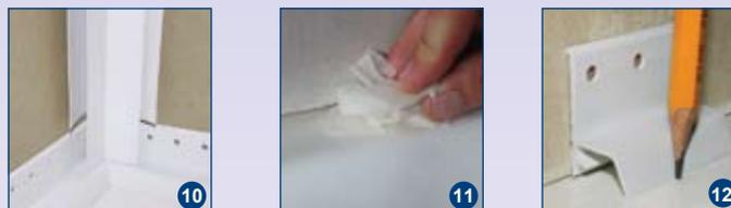
11. Wipe ledge with alcohol wipes. 12. With pencil and small strip off-cut, lightly mark where strip outer edges rest on ledge (4 points/side).
