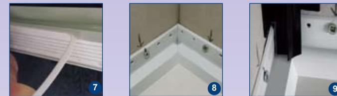
8-10 8. An adhesive fixing of the strips to the wall (17-18) may be strengthened with a mechanical fixing (screw/nail) if the weight of the wall panels is likely to dislodge freshly adhered strips because the adhesive/sealant has yet to cure. This is not an issue where panels are supplied in the form of lengths but to be considered if wall panels are supplied in sheets. 9-10. If corner trims are being installed, notch corner trim flanges so trim end rests on strip.
