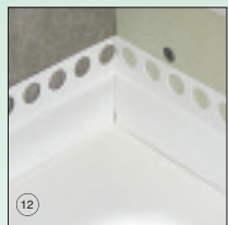
12 Ensure Sealux-N fuses across joints inside strips
