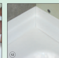
12 Ensure Sealux-N fuses across joints inside strips
