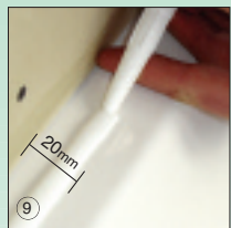
9 Lay a line of Sealux-N on ledge using finger as guide
