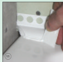
11 Remove excess Sealux-N on ledge (if any)
