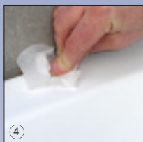
④ Clean ledge using Sealux alcohol/meths wipes
