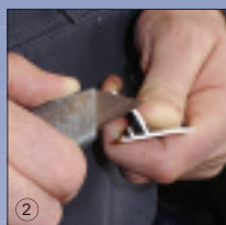
② Carefully remove frays left by saw cut!
