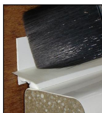
**Solution:** This task is made easier and quicker by first installing a Sealux Reg 20 profile over the joint, masking the strip and dressing the membrane down over the up-stand.
