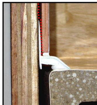
**Solution:** The installation of Sealux Reg 20 can bridge wall/ledge gaps up to 12mm. This makes waterproofing possible over all shower trays and baths.
