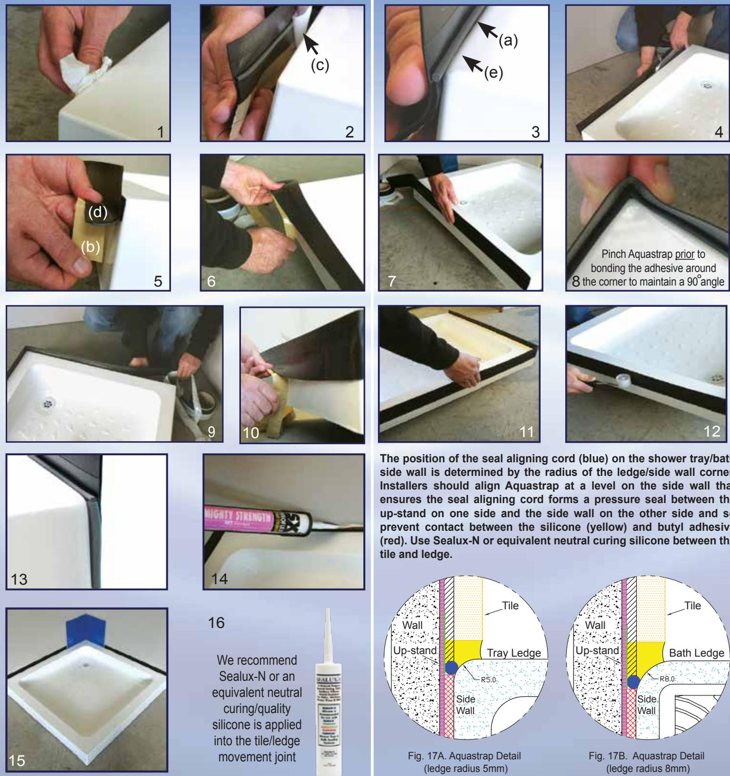
The position of the seal aligning cord (blue) on the shower tray/bath side wall is determined by the radius of the ledge/side wall corner. Installers should align Aquastrap at a level on the side wall that ensures the seal aligning cord forms a pressure seal between the up-stand on one side and the side wall on the other side and so prevent contact between the silicone (yellow) and butyl adhesive (red). Use Sealux-N or equivalent neutral curing silicone between the tile and ledge.
